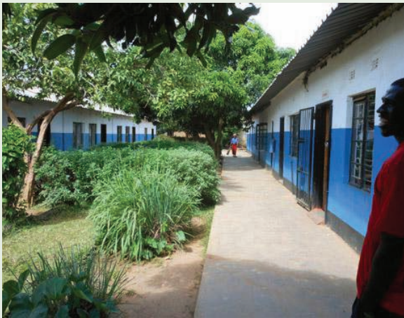
© Schoollinks Classrooms at Buyantanshi Open Christian Community School
